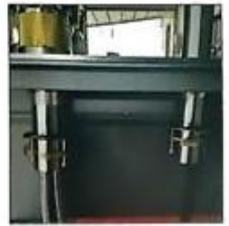
3: Insert the two water inlet pipes into the faucet, pay attention to the position of the hot and cold water pipes
