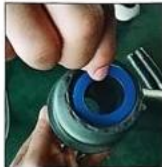
10: Put the sealing ring on this pipe joint
