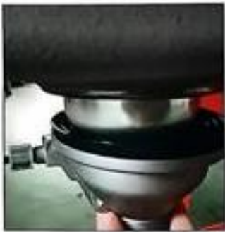
4: Put the drainer into the circular opening of the sink and tighten it
