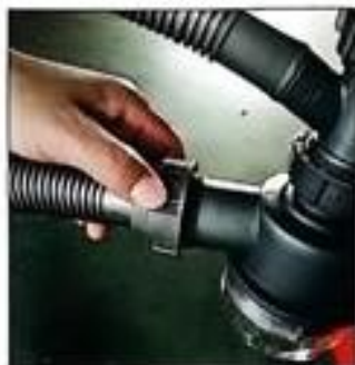
12: Put the silicone sealing ring on the connection with our sewage pipe, and tighten the hose main pipe
