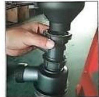
11: Fix the sewer pipe and connect to the sewer system
